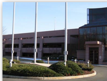
UPS 340 MacArthur Blvd Mahwah, New Jersey
