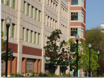
Montclair Parking Authority Montclair, New Jersey
